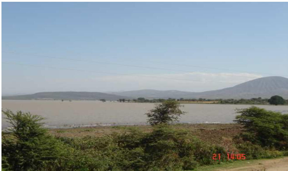
Photo 1: Partial View of Koka Dam (Abiyu, 2007)
